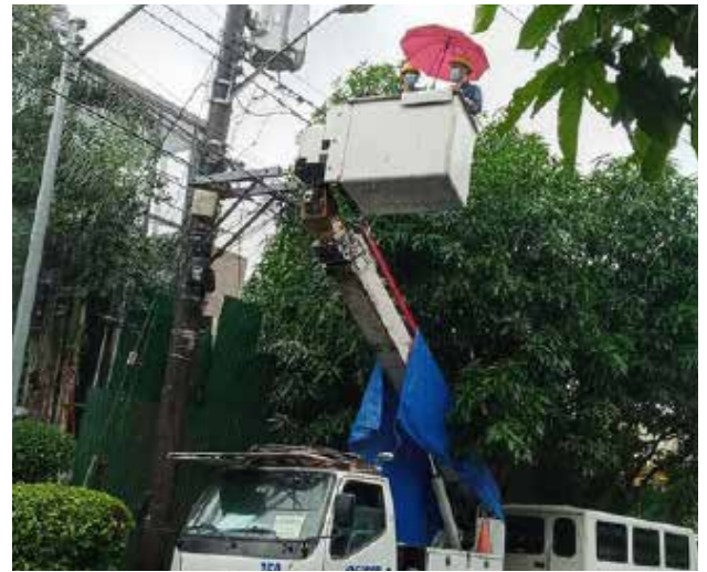
Repair of busted lights and lamp post
