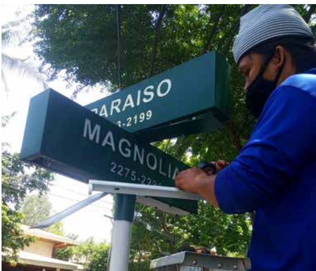
Repair of Lighted Street Name
