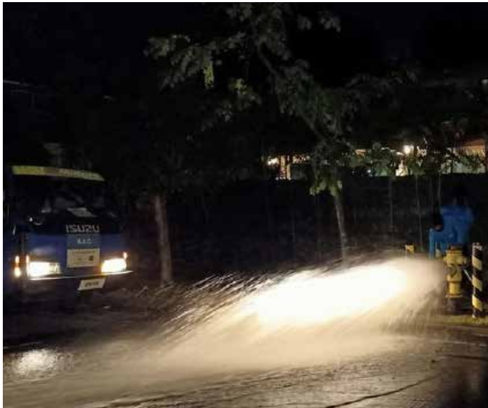
Rehabilitation of Dasma Deepwell
