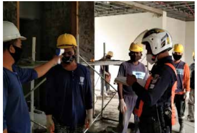
Thermal Scanning at the jobsites
