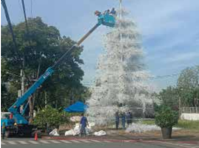
Installation of 30ft Christmas Tree
